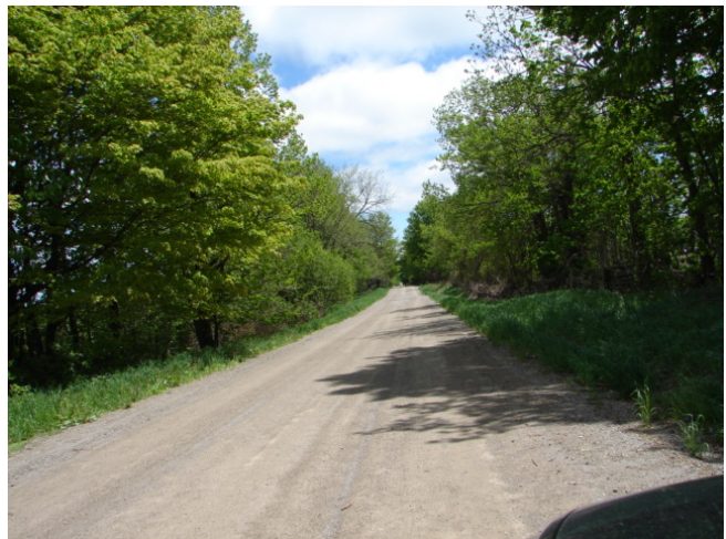
Photo 3 – Sixth Line looking south
