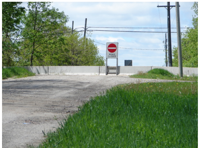
Photo 18 – Sixth Line dead ends at the north at railway right-of-way
