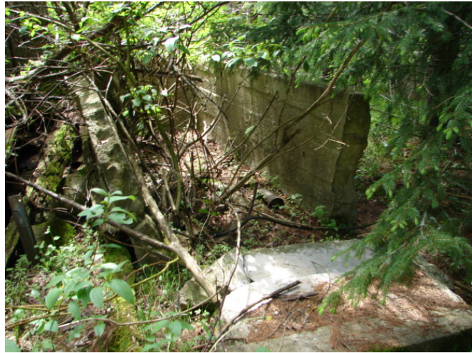
Photo 7 – Concrete cistern at farmhouse site
